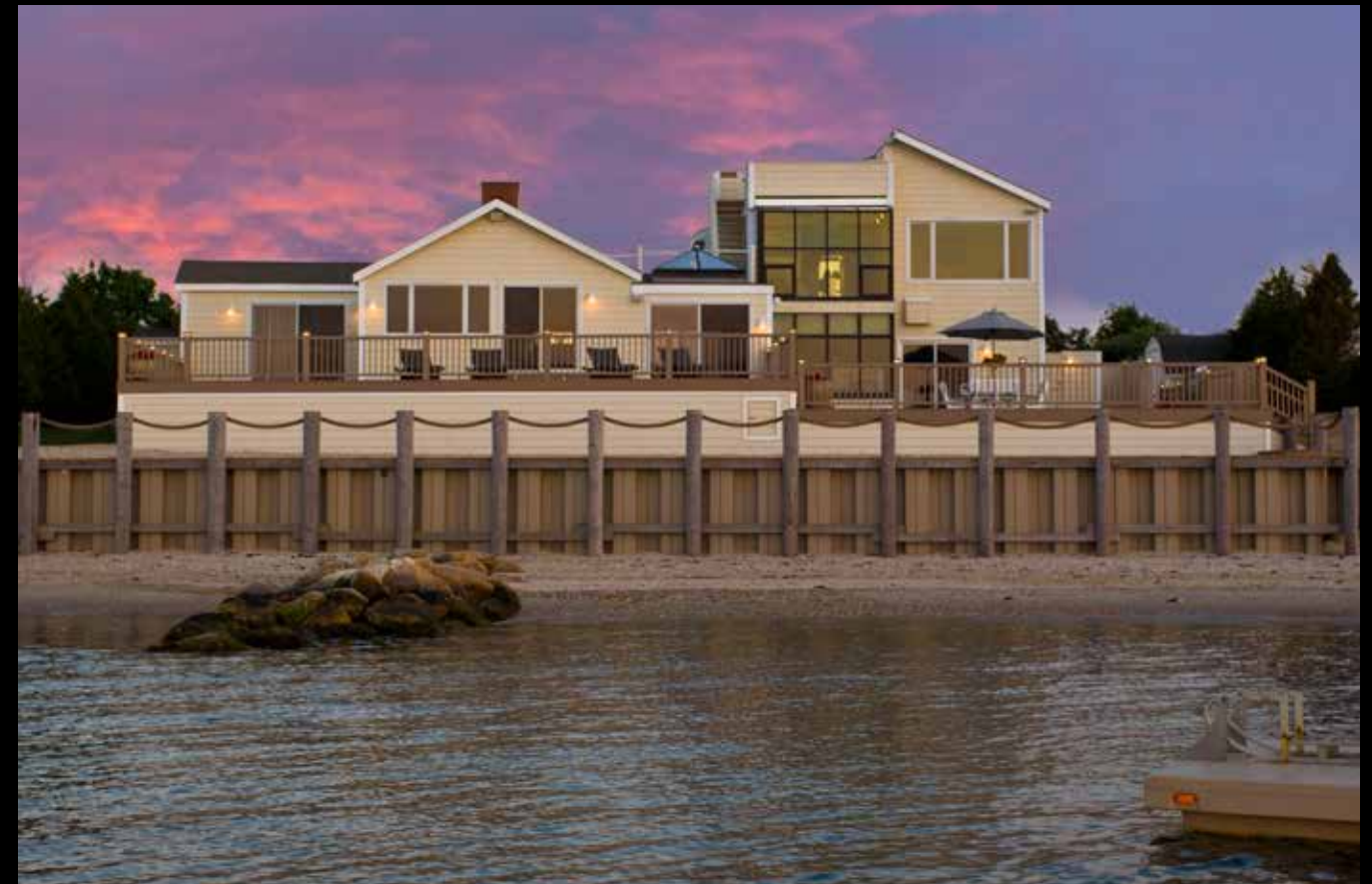
Rear Exterior View from Gardiner's Bay
