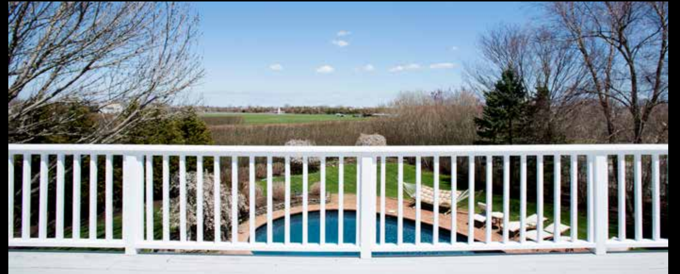
2nd Floor Terrace
